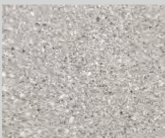
Exposed Aggregate finish
