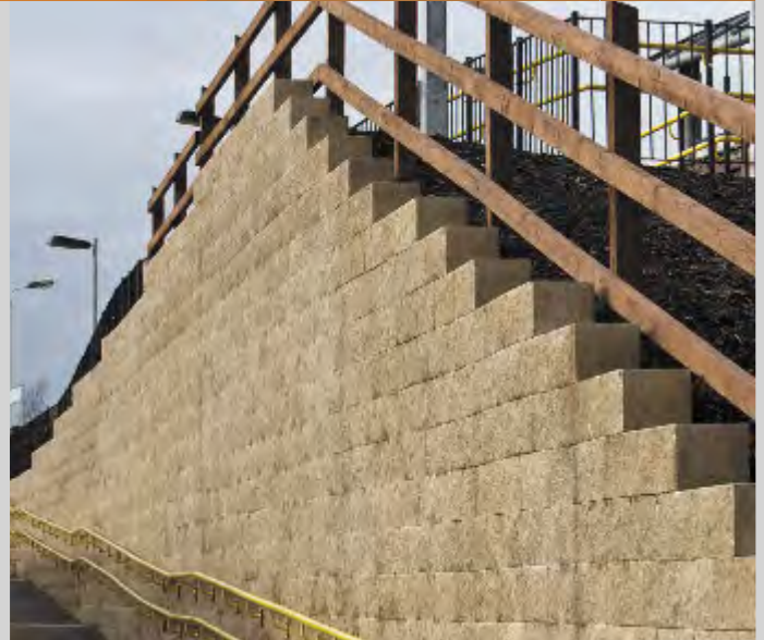
Passenger access, Littleborough Station, Rochdale
